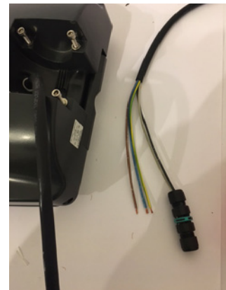
STEP 8 Wire the dimming cores into the central free connector keeping colour as in the picture.
